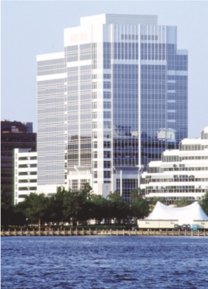
The 150 West Main Tower provides ten stories of Class A office space and ten stories of parking at the gateway to Norfolk's financial district.
